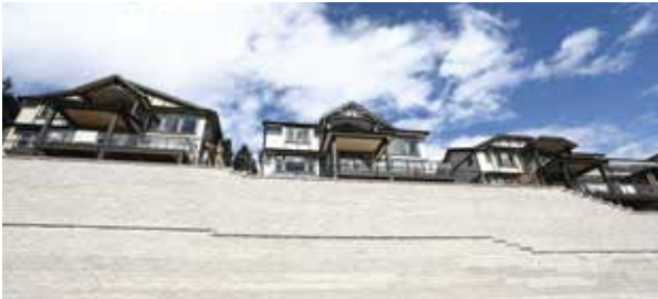
Large Retaining Wall Projects
