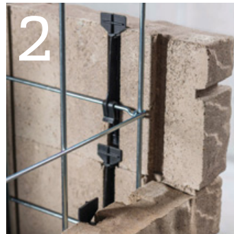
Use connector to attach veneers to grid
