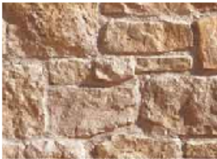
Wheatfield Rough Cut with an overgrout technique
