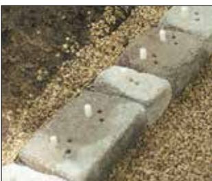
3. Insert Fiberglass Pins
