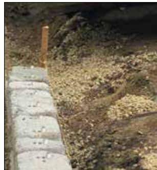
4. Install Fill & Compaction
