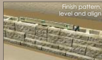
Compact on block and behind
