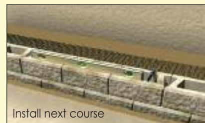
Install AB Reinforcement Grid
