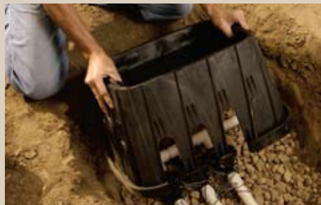
Reattach the knock-outs to keep out backfill dirt.
