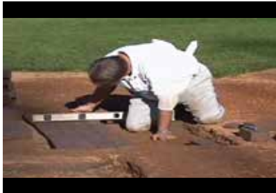
Renovating Batter's/Catcher's Boxes 2:54
