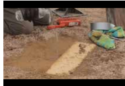
Mound Hole Repairs with Clay Blocks 1:17
