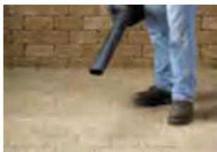
Wetting should take place in sections at a time: **RG+**: 200 sq. ft (20 m<sup>2</sup>), **HP**: 500 sq. ft (50 m<sup>2</sup>). Ensure that the wetting of one section is finished before another section is started.
