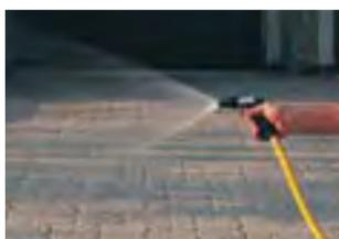
Produce a very fine mist so that the water falls gently without displacing the polymeric joint. Moisten the whole section lightly and in a continuous manner; avoid flooding the surface and causing runoff. Using a small screwdriver, verify the progress of the wetness in several areas by emptying a small portion of the joint. Once the joints are moistened 1.5" (4 cm) deep, stop watering the section and move on to the next one.
