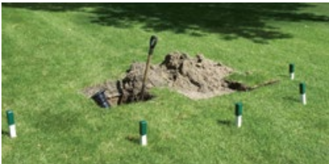
Mark off repair areas.
